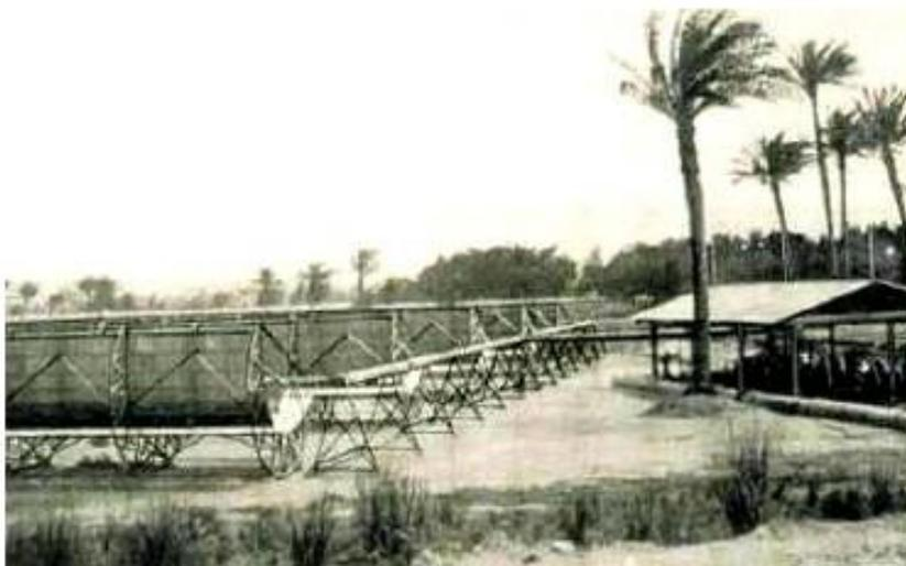
*First parabolic trough collector developed by American inventor Frank Shuman in Cairo (1912)*
